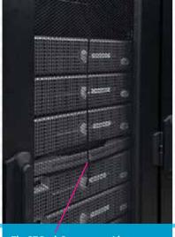
The 2T Rack Sensors provide two temperature readings per rack. A single Liebert CRV reads the sensors for up to 10 racks.
